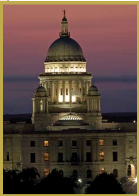
The RI State House was designed in 1892 by the legendary New York architectural firm McKim, Mead and White. Made of white Georgia marble, it has the fourth largest self-supporting marble dome in the world.
